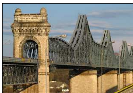
Fig. 9. The Anghel Saligny's Bridge
